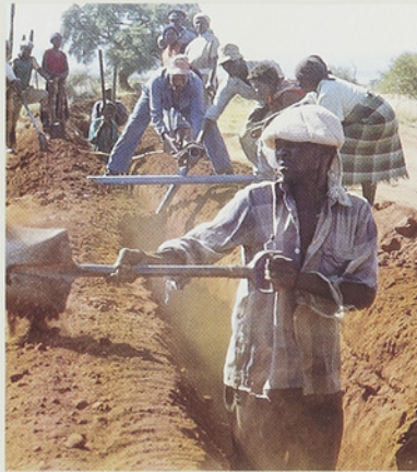
Villagers from Mabeskraal line trenches with soft soil to accommodate the trunk mains that will bring water to their village in arid northern Bophuthatswana.
